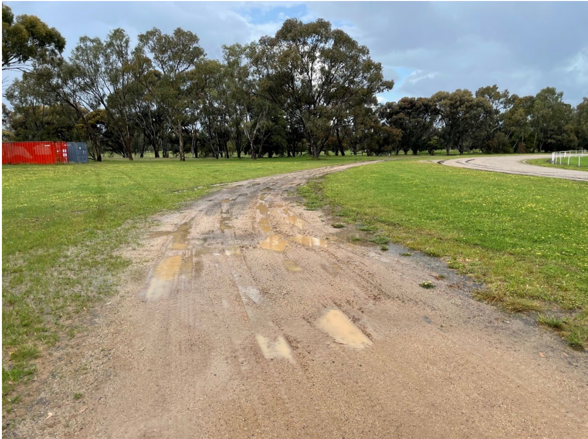
Image 3: Bog holes on tracks near the trial site in Numurkah Showgrounds
