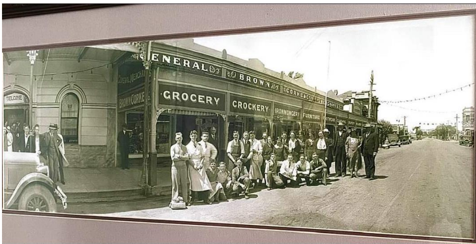
Image 10: Early image (1920's?) shows the site as a series of buildings with decorative facades, individual shopfronts and ornamental skillion verandah. The front wall is aligned with the front wall of the Telegraph Hotel.
