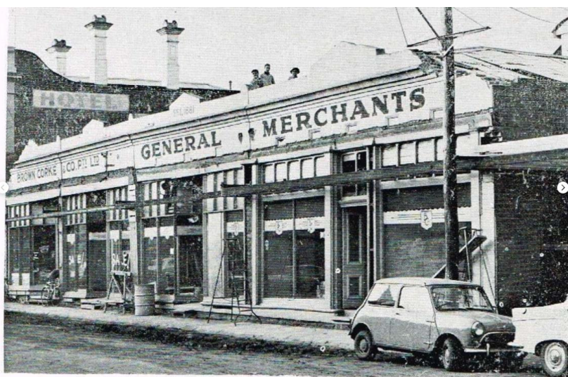
A FACELIFT FOR BROWN & CORKE'S IN 1964. A. J. Pumba. Photo.
