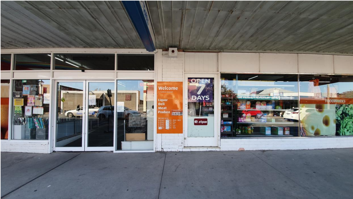
Image 15: Existing front presentation to Melville Street, shows remnants of the 1960's alterations typical to changes made to buildings within the streetscape with the introduction of expanses of wall and glazing.
