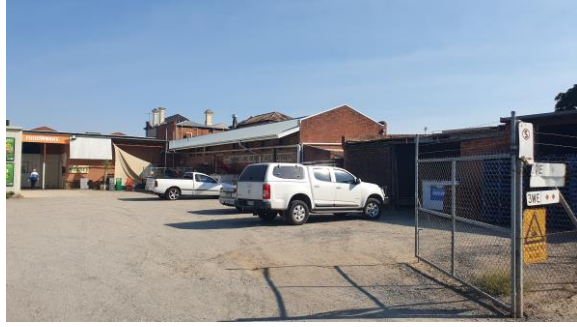
Image 18: View to the rear showing informal layout of the carparking and delivery area together with the outbuildings and storage area.
