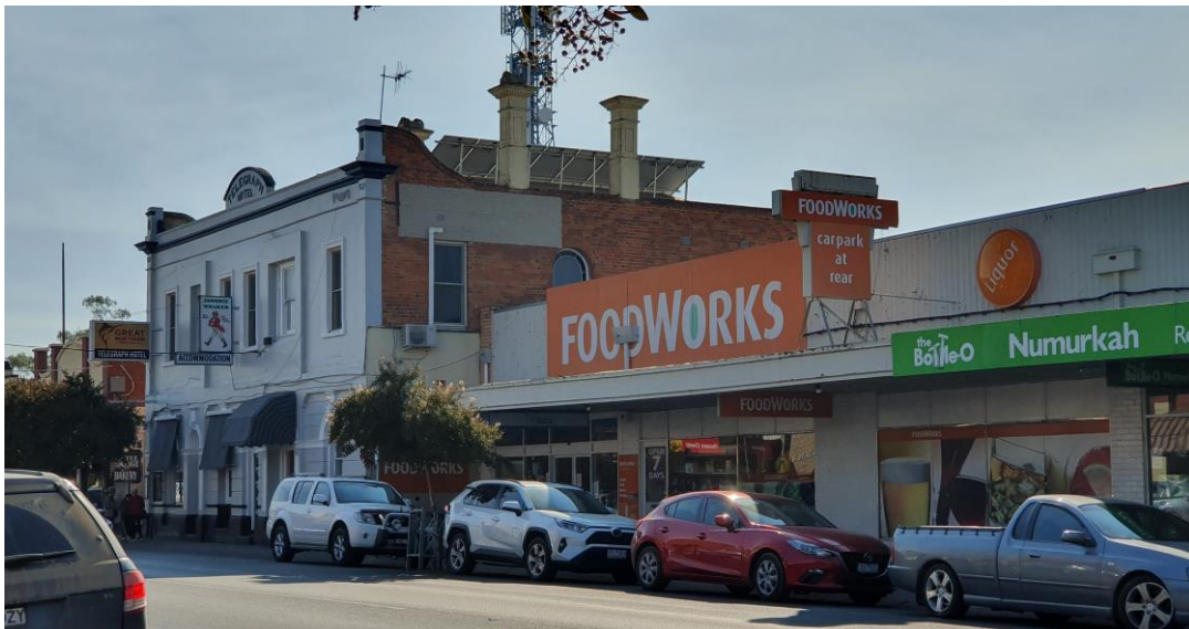
Images 4, 5: The Telegraph Hotel (1882) is historically significant as the oldest hotel in Numurkah. The abutting FoodWorks building as a single storey building is lower in height which is consistent with the earlier contributory buildings on the north side of the Hotel. Uniformity in the overall façade and parapet height to both sides of the Telegraph Hotel allows it to have visual prominence within the Streetscape.
