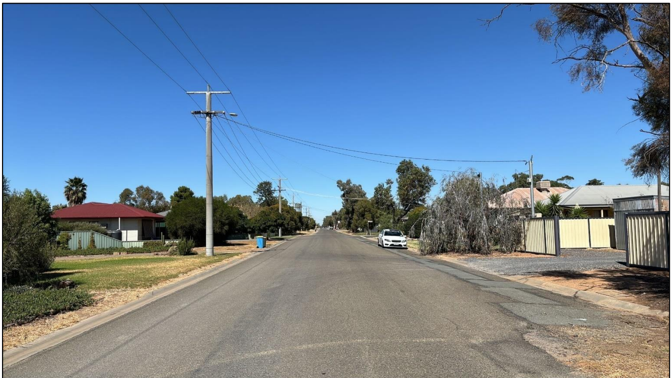
Figure 6: Katunga North Road facing south
