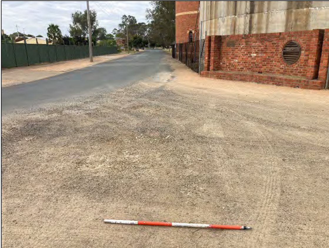
Photo 8: Site conditions near old water tank off Gray St, imported gravel fill. Good (Gravel) to Zero (Asphalt) GSV. Photo: D.Wall, 2023.
