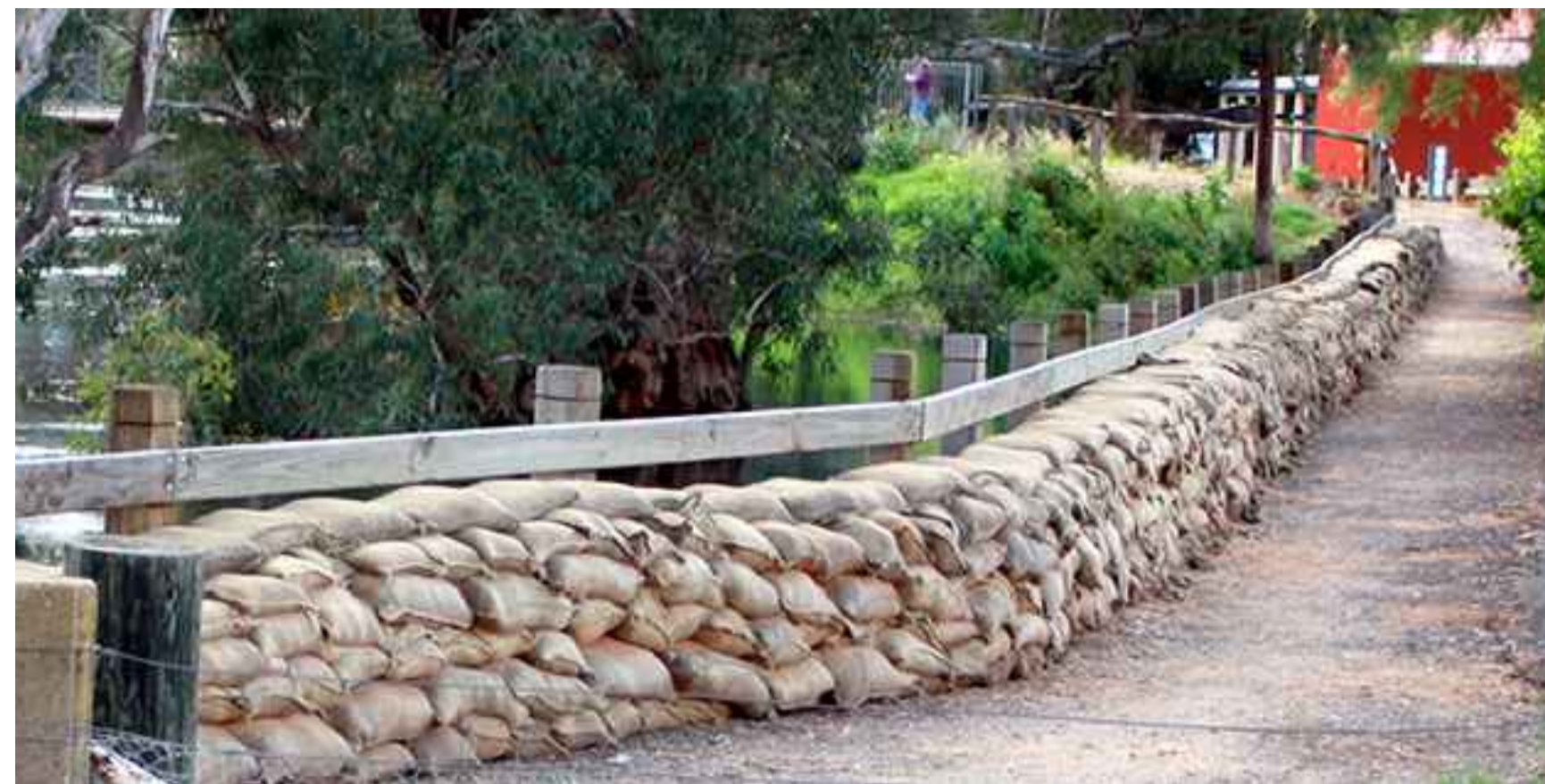
TYPICAL TEMPORARY SANDBAG LEVEE NOT TO SCALE
