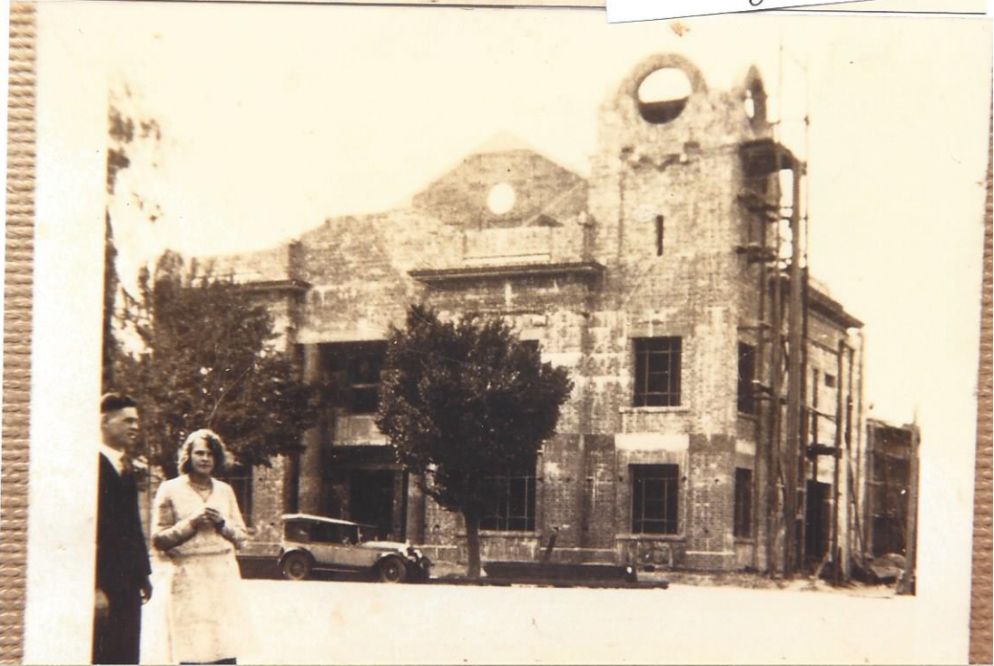
5/4 1930 Building the Shire Hall
