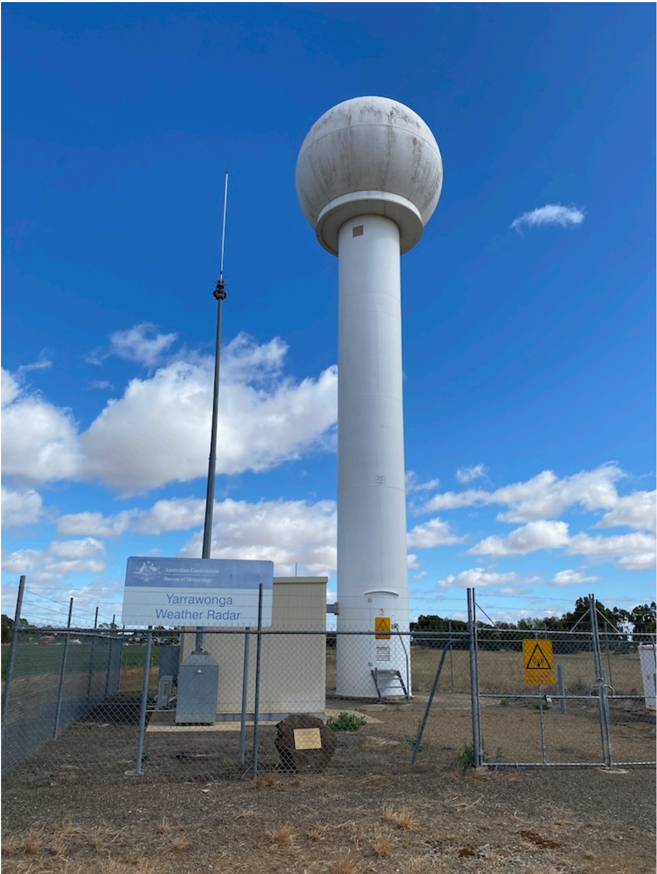
BOM Radar Station
